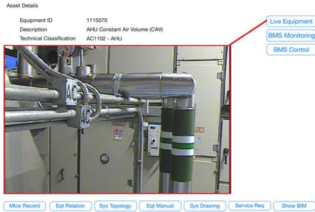
Figure 6: CCTV live feed in the BIM-AM System at the mobile terminal
